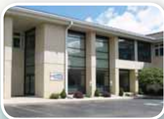
Main Office in Muncie
